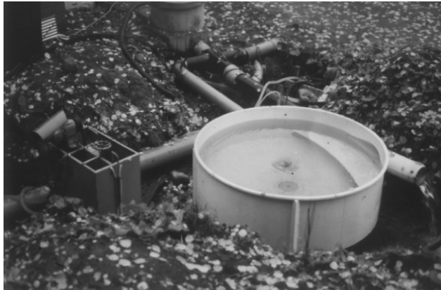
Figure 10: Swirl concentrator Fish Hatchery facility in Lammi, Finland, summer 1986 (Mashauri, [2])
