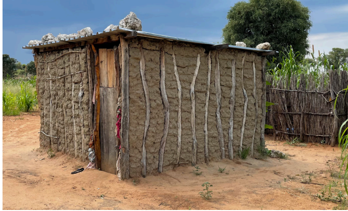
Figure 50: Traditional clay house with mono-pitched corrugated iron roof with rock weights.
