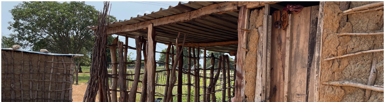
Figure 110: Homestead kitchen wooden frame structure allowing light and air to pass through
