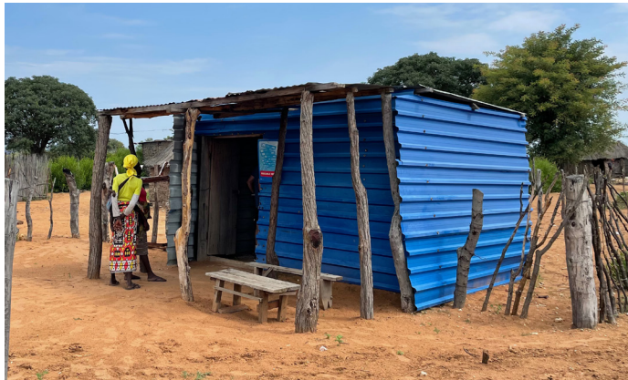
Figure 52: Corrugated iron structure.
