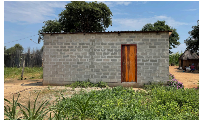
Figure 26: Cement brick housing typology.
