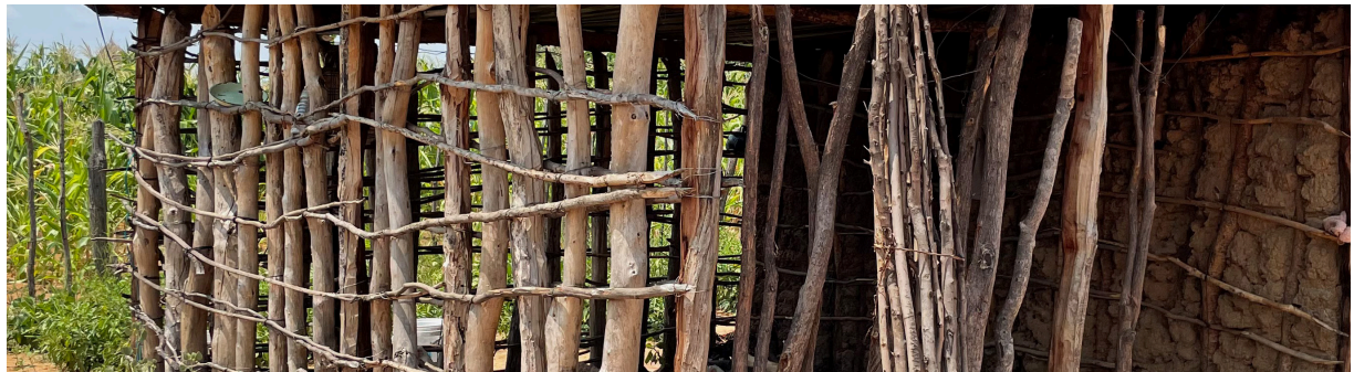
Figure 105: Homestead kitchen with an exposed wooden frame structure
