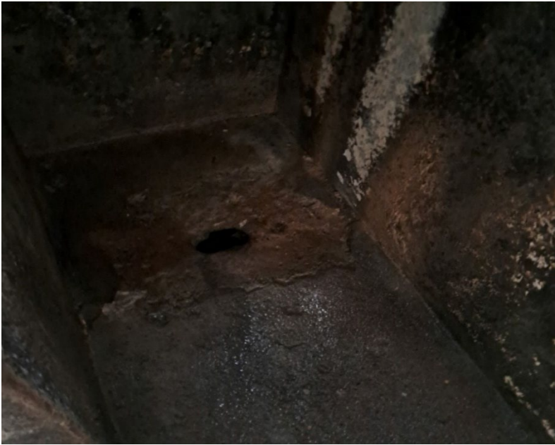
Figure 4: Shower Cubicle, Police Station, Windhoek Central
