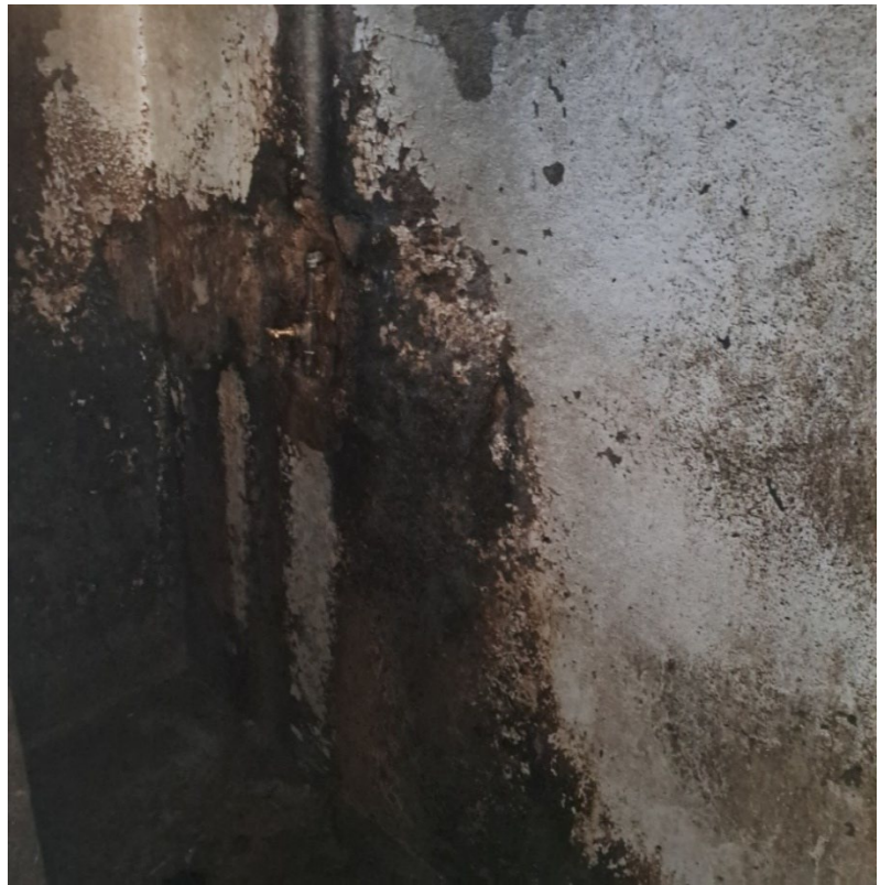
Figure 5: Shower Cubicle, Police Station, Windhoek Central
