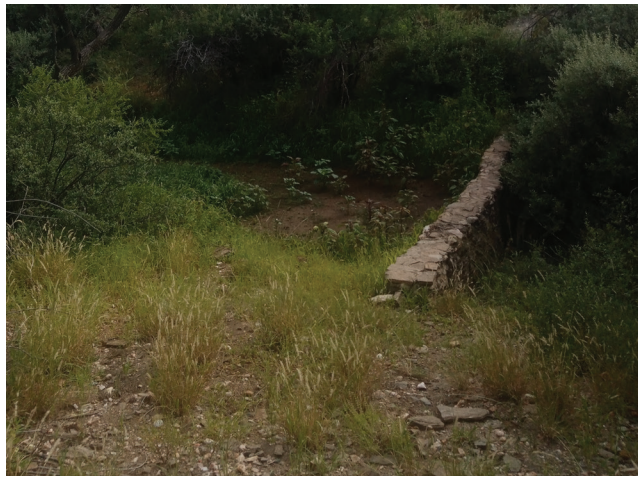
Figure 101: A dam wall at the bottom of the valley to keep water in as long as possible
