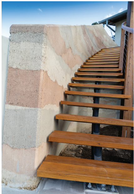
Figure 85: A photo showing the aesthetic qualities of a rammed earth wall (Rammed Earth Constructions, 2023)
