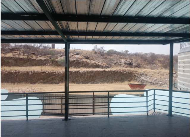
Figure 118: The hole as seen from inside the cafeteria
