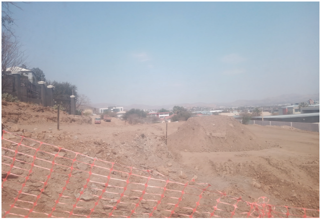
Figure 22: Example of site scraping
