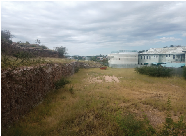
Figure 117: A photo showing just how steep the cuts are into the site
