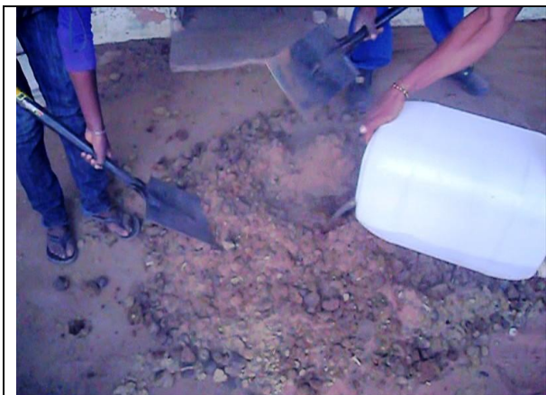
Water is added to mix with cow dung and soil.
