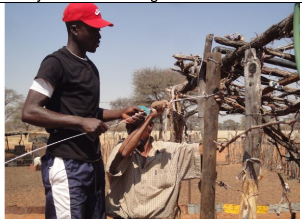
A stay wire is secured.
