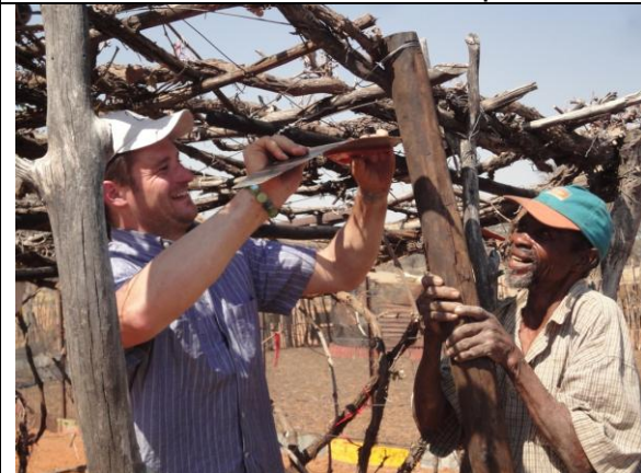
A new pole is secured.
