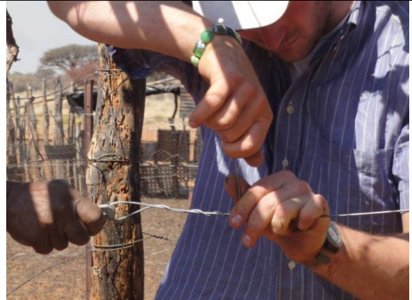
... Even its poles are rotting.
