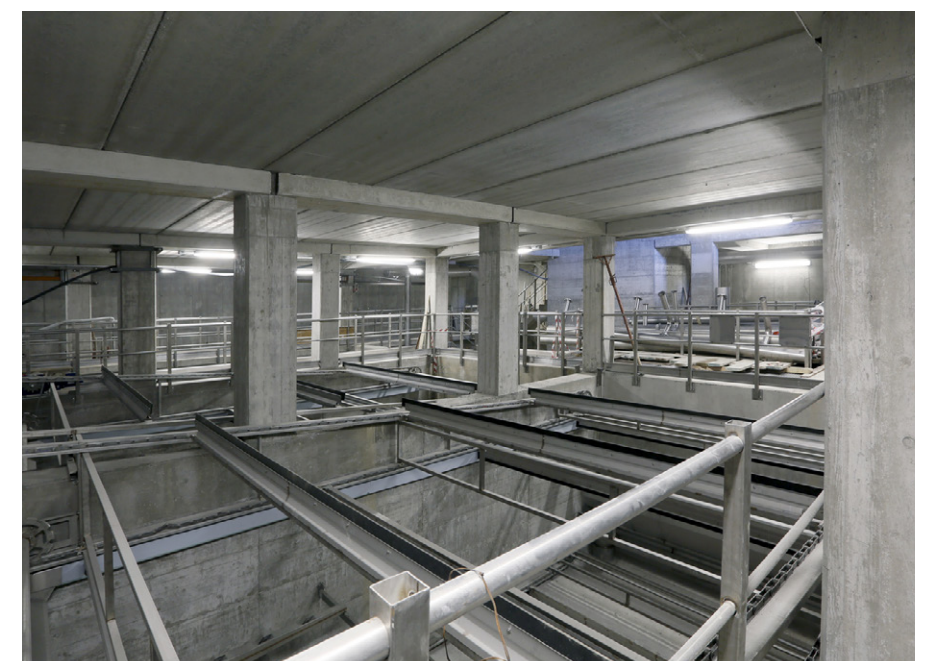
Figure 44: Photo of treatment area (Archdaily, 2016: online.).
