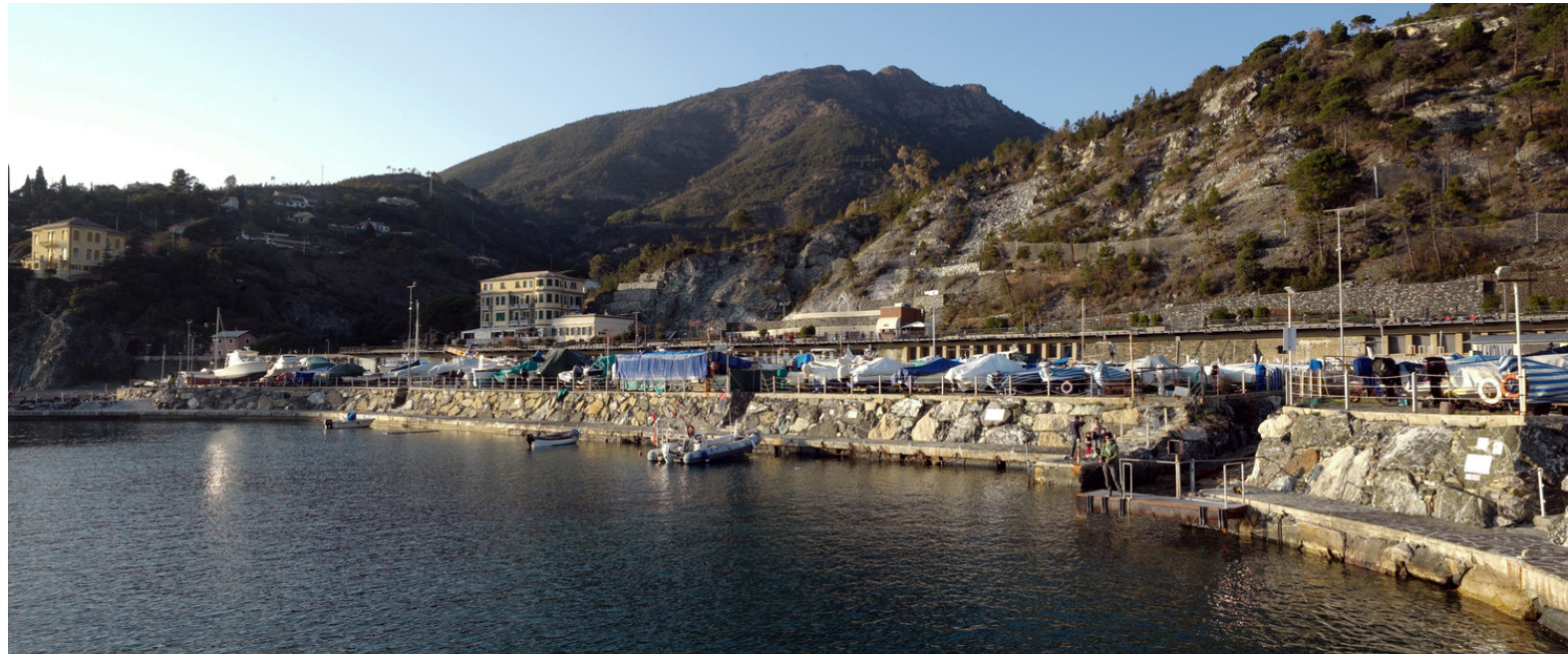
Figure 41: Photo from water (Archdaily, 2016: online.).
