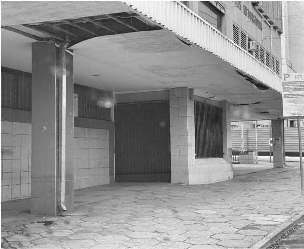
Existing building entrance on Independence Avenue, entrance closed off to public after home Ministry of Home Affairs moved out of CBD.
