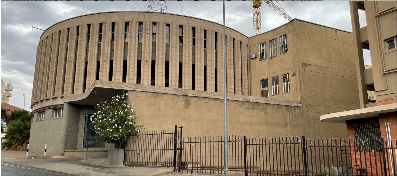
Figure.59c: Cohen Building view of Radio Tower from Fannie K. Street.
