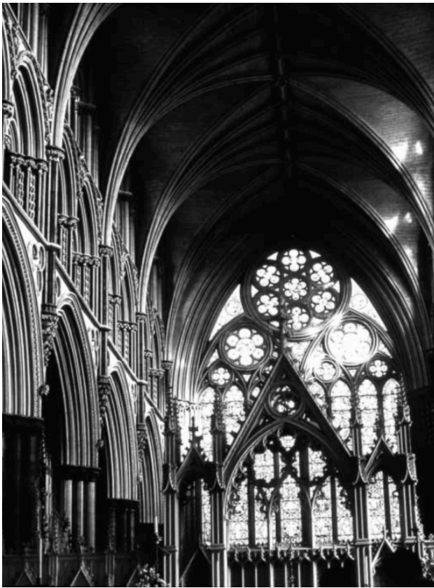
Figure.44b: Lines within the Lincoln Cathedral. Source: Hardy, A. (2011). The expression of movement in architecture. The Journal of Architecture, (Issue 4), 471–497. https://doi.org/10.1080/13602365.2011.598698
