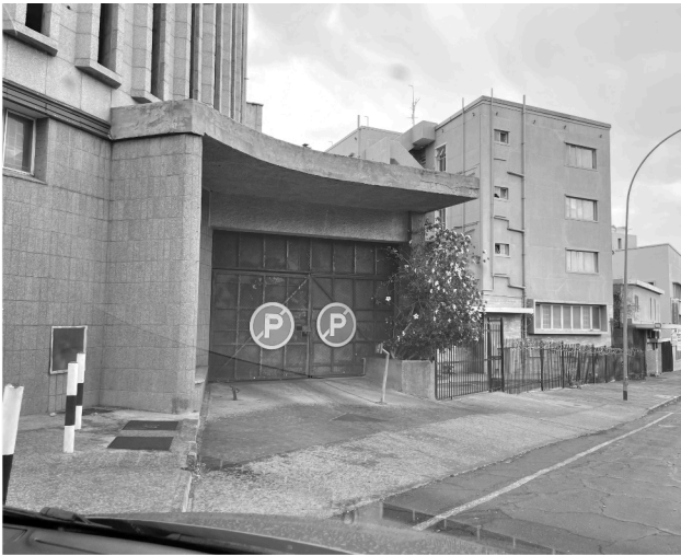
Existing building entrance on Fonniesburg Road, mainly for vehicular access to the building ramps.
