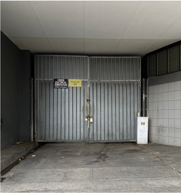
Figure.52a: Photo of closed-off path through alleyway
