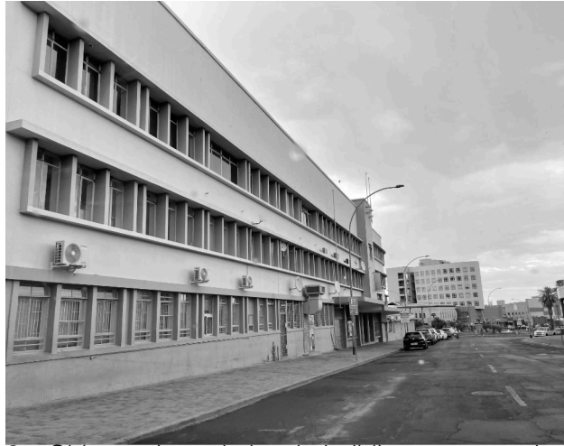
2. Old continental hotel building, unoccupied building in the CBD area.
