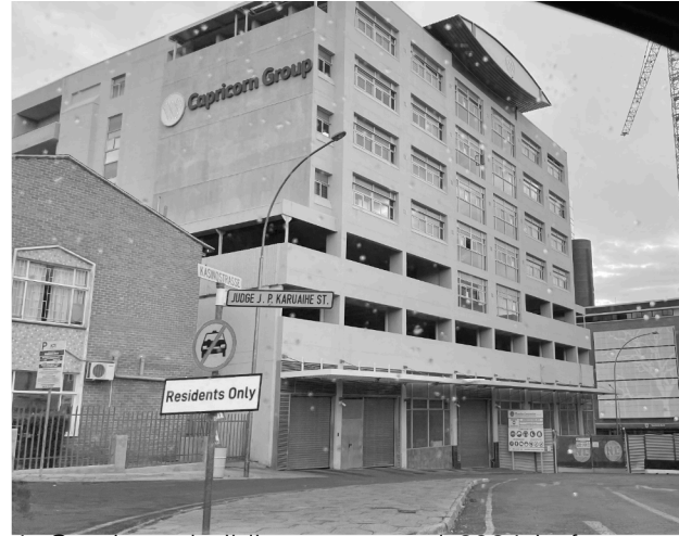
4. Capricorn building evacuated 2024 in favour of new headquarters outside of CBD area.
