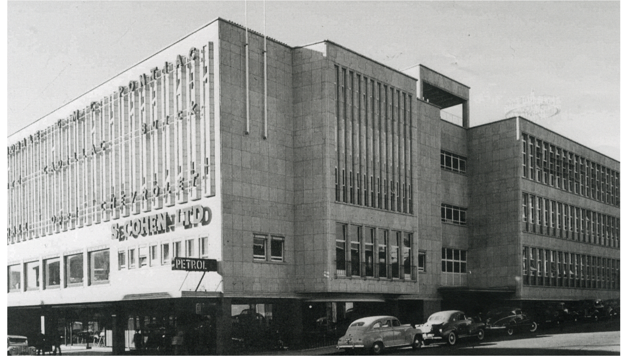
Figure.57: Cohen Building after Completion. Source: Gill, F. (Ed.). (1956). Cohen of South West Africa. South West Africa Commercial Holdings Limited.
