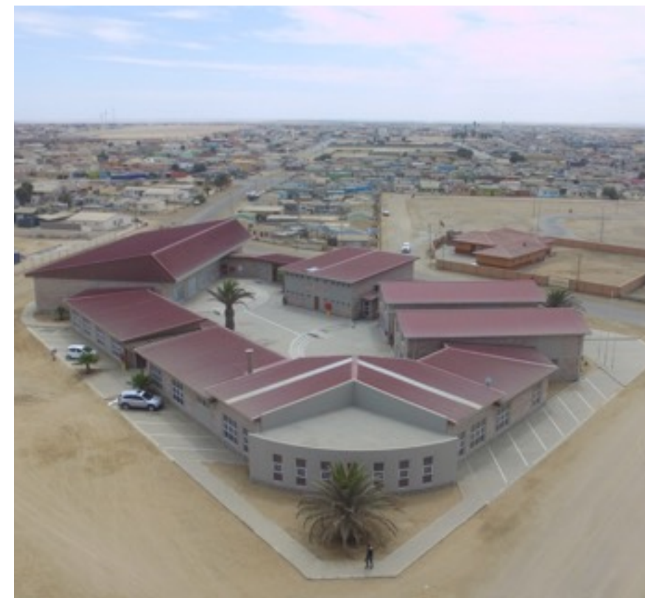
Figures: Overview of the Mondesa Multi-purpose Centre.
