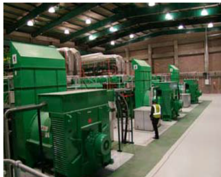
Figure 1.1: Anixas Power Station: Oil-fuelled generator sets.
