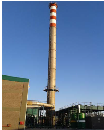
Figure 1.3: Anixas 60m high cluster exhaust stack
