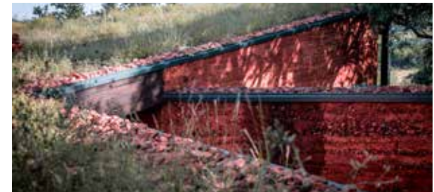
Figure 2.3.2 - Witklipfontein Eco Lodge - Rammed earth walls to absorb heat reducing interior heat gain
