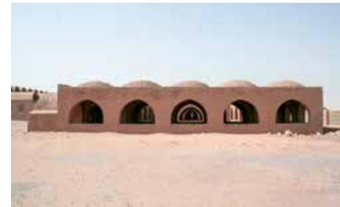
Figure 2.4.2 - New Baris Village - Deep spaces to shade and cool interior Image by Senses Atlas (2020). https://www.sensesatlas.com/hassan-fathy-building-in-the-desert-in-new-baris/
