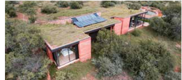
Figure 2.3.1 - Witklipfontein Eco Lodge - South facade with views to each space and access to natural sunlight
