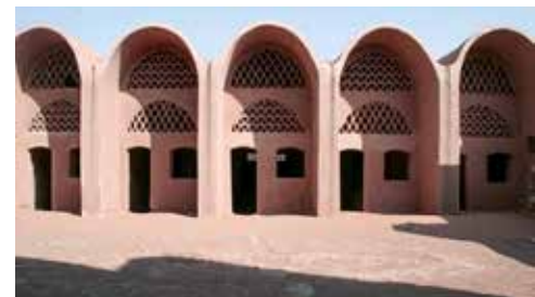
Figure 2.4.3 - New Baris Village - Facade setback with fenestration cool and vent heat interior Image by Senses Atlas (2020). https://www.sensesatlas.com/hassan-fathy-building-in-the-desert-in-new-baris/
