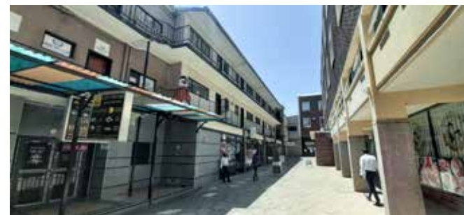
Figure 5.1.15 - Thoroughfare / arcade between buildings
