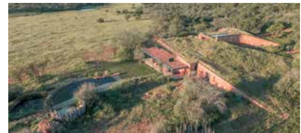
Figure 2.3.3 - Witklipfontein Eco Lodge - Building set into landscape utilising earth edges to cool interior spaces
