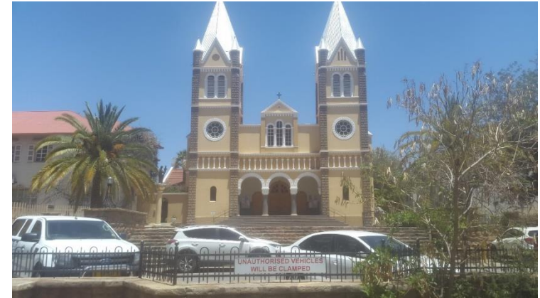
Fig 4.2: Roman Catholic CBD Romanesque Revival Architecture church building (Author 2021).
