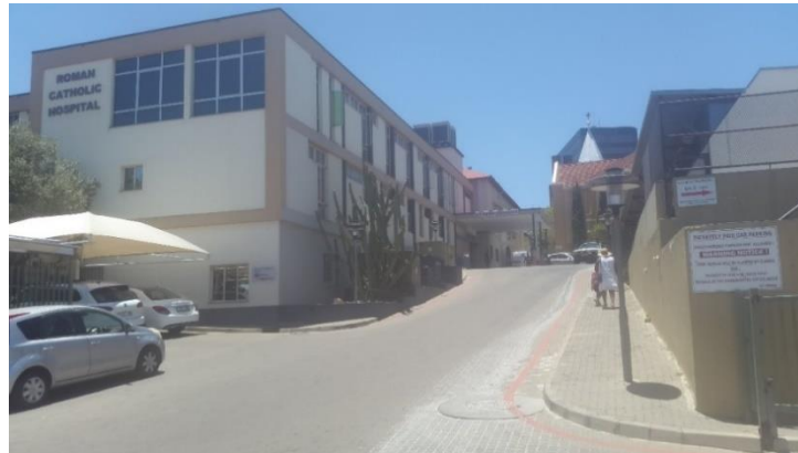
Fig 4.3: Roman Catholic Church CBD photo showing the recently extended hospital from the western side (Author 2021).
