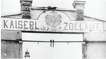
Figure 1.56 Demolished Customs Shed
