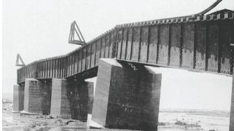
Figure 1.58 Railway Bridge crossing Swakopmund River
