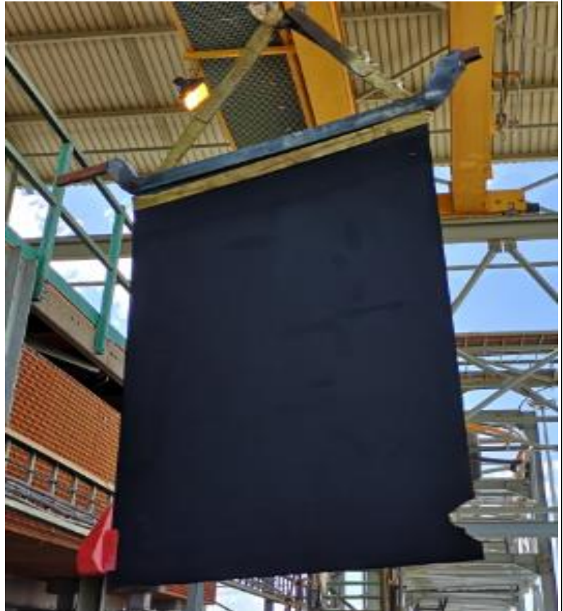
Figure 4.50: An anode with a missing side insulator (picture taken by the author)
