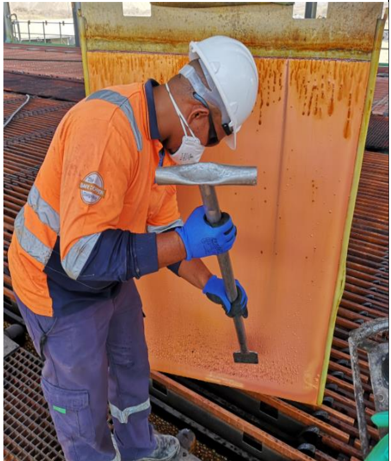
Figure 4.52: Knocking off nodules that caused a hotspot (picture taken by the author)
