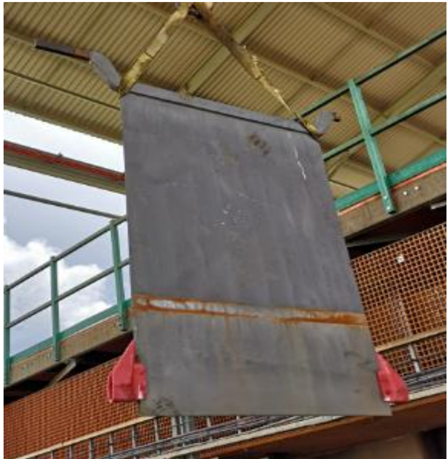
Figure 4.54: Hoisting up a new anode (picture taken by the author)
