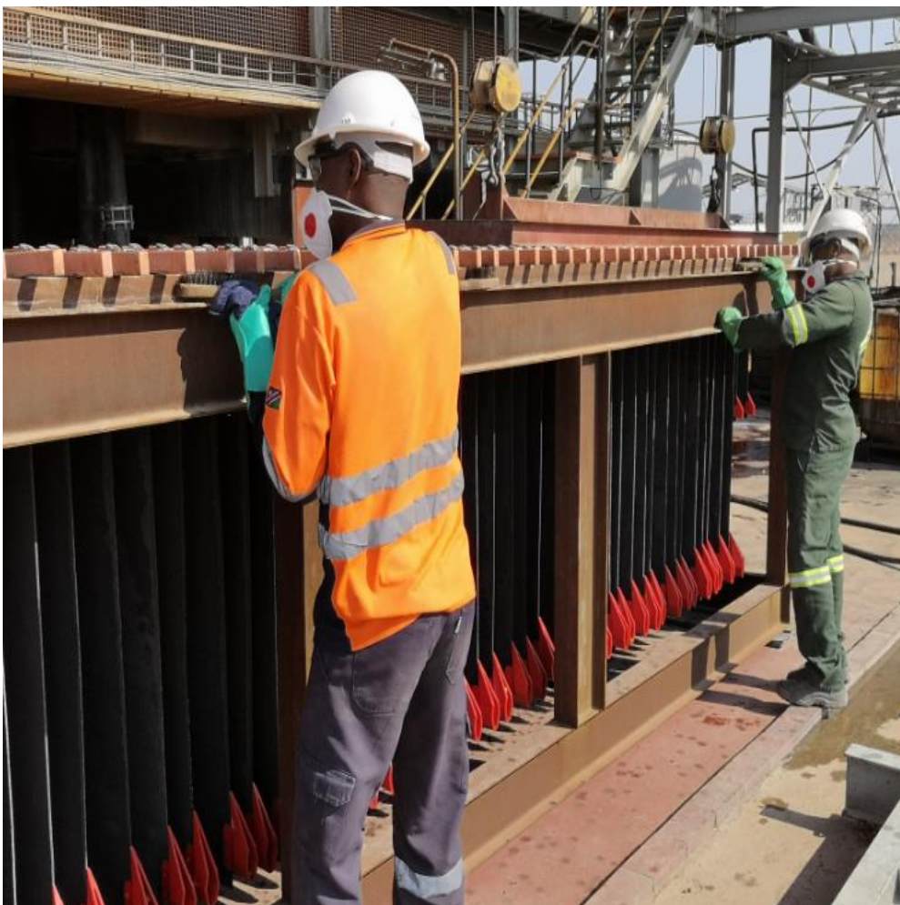
Figure 4.26: Cleaning anode contacts using steel brushes (picture taken by the author)
