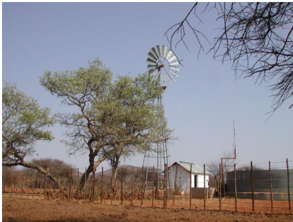
Wind energy is used to pump water at most of the Queen Sofia boreholes.
