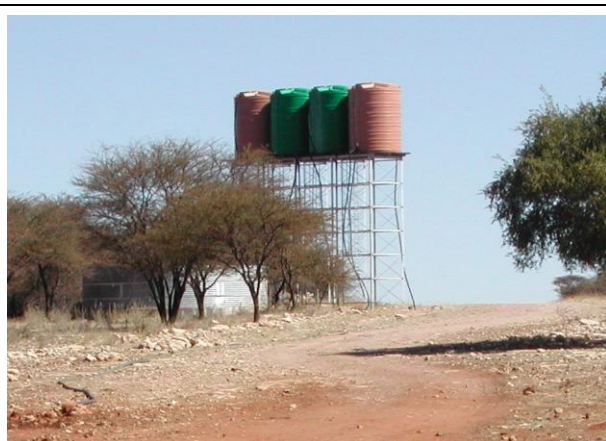
The capacity of the four tanks that supply water to the fifty homes and school comes to a total of 40m 3 .
