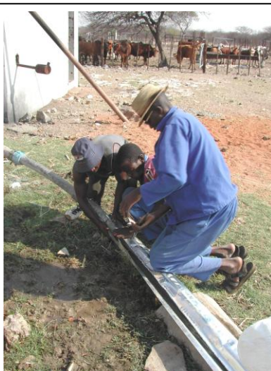
The polypipe that got damaged by a porcupine gets protected with a covering of galvanized sheeting.
