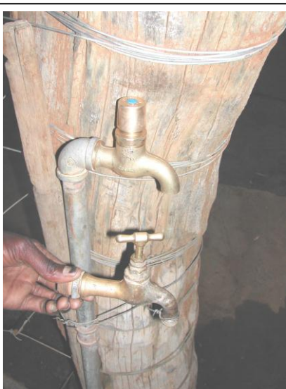
The screw tap, below, was replaced with a push tap at the school, to save water.
