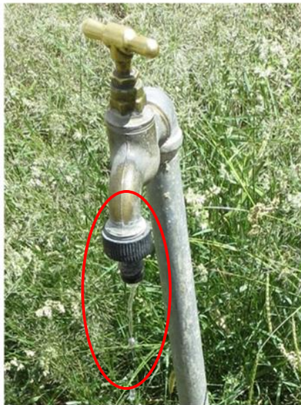
Figure 7: Examples of leaks detected during the April 2020 lockdown.
